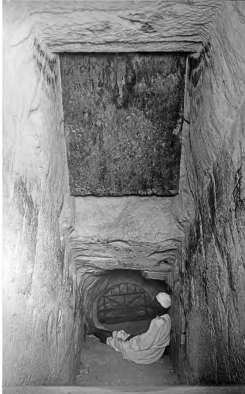
The Descending Passage of the Great Pyramid of Gizeh ; the lower reach of which is now closed by an iron grill door ; showing the lower butt-end of the Granite Plug in the roof. The Granite Plug closes the entrance of the First Ascending Passage
