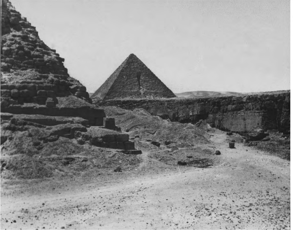
The north side of the THIRD PYRAMID of Gizeh : showing the deep chasm excavated by the Mamelukes in their search for the Entrance of the pyramid ; also the north-west corner of the Second Pyramid ; with part of the artificial cliff to the west, formed by the ancient builders in their rock-levelling operations
