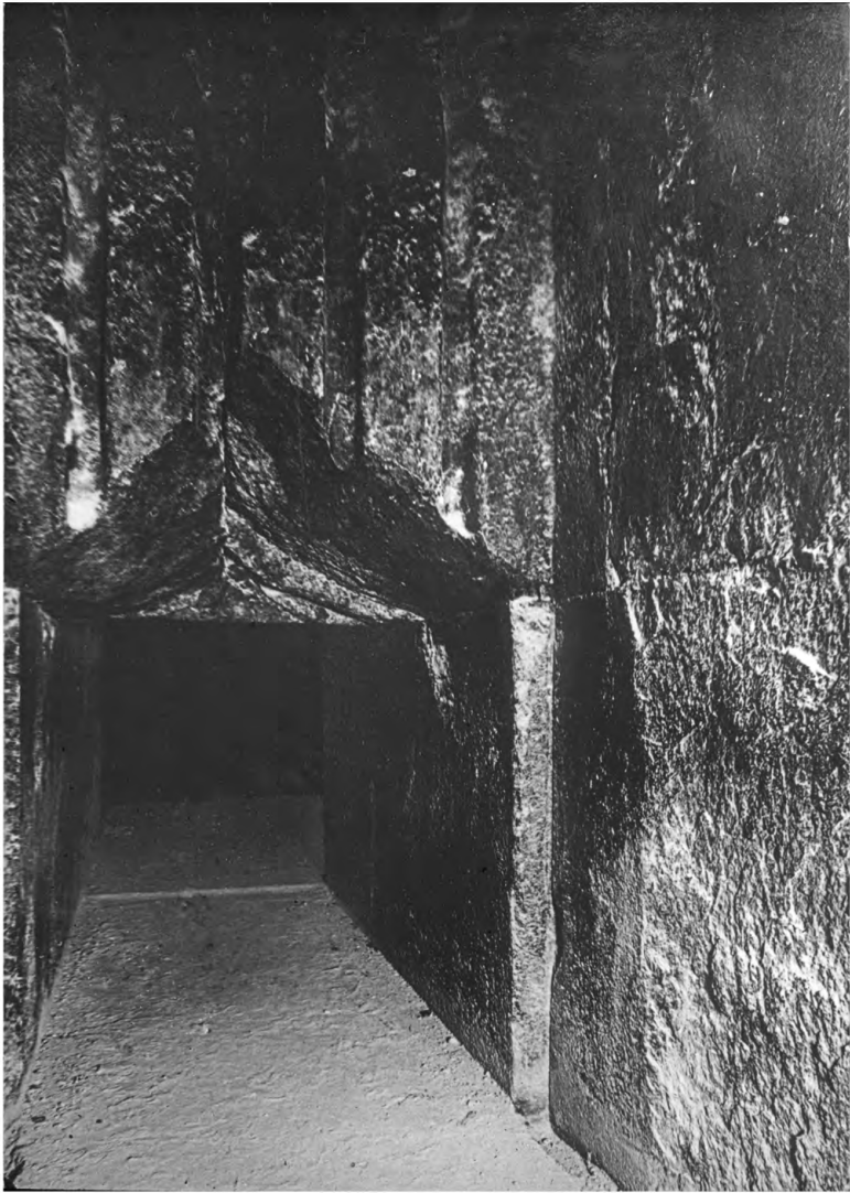
The south wall of the ANTE-CHAMBER; showing the four deep grooves which divide the wall into five equal spaces; also the low passage which leads southward to the King's Chamber—Compare with Plate XXXV
