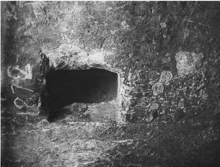
The north air-channel of the Queen's Chamber ; showing part of the five-inch thickness of once-concealing stone
