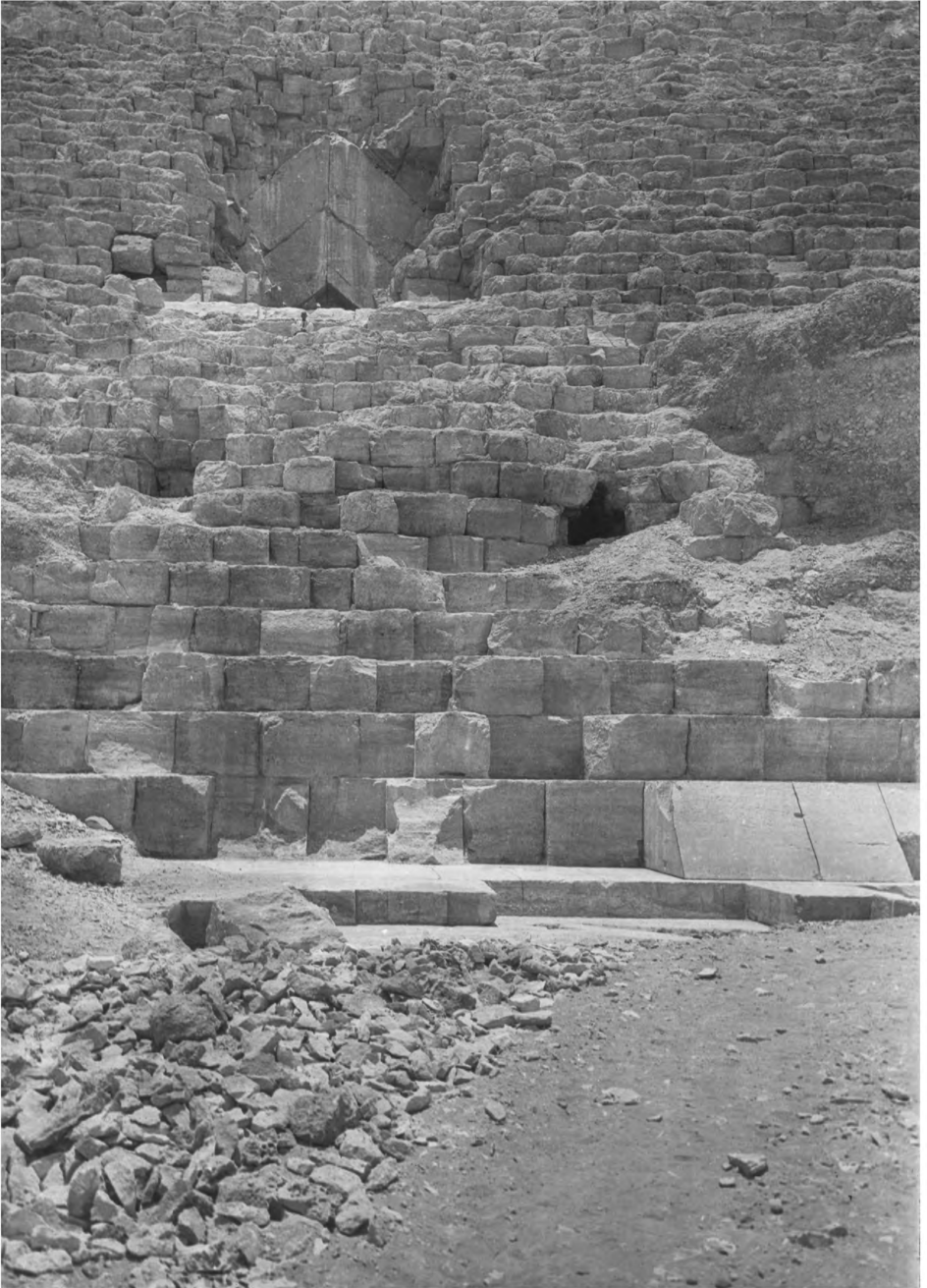
The MIDDLE of the NORTHERN SIDE of the Great Pyramid of Gizeh ; showing angle-stones above the entrance, and the casing-stones
