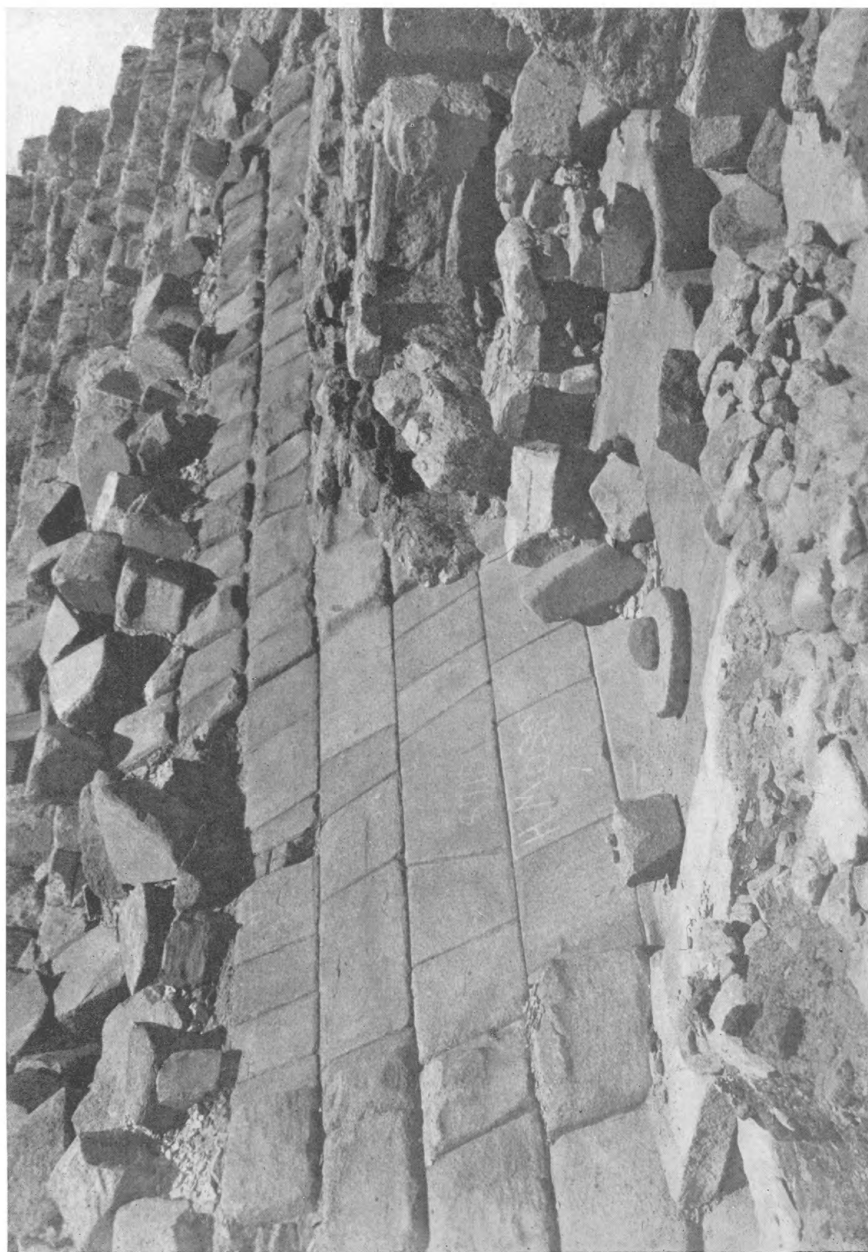
The east base of the THIRD PYRAMID of Gizeh; showing partly dressed granite casing-stones still in situ; also a portion of the granite pavement of the Pyramid's temple.
