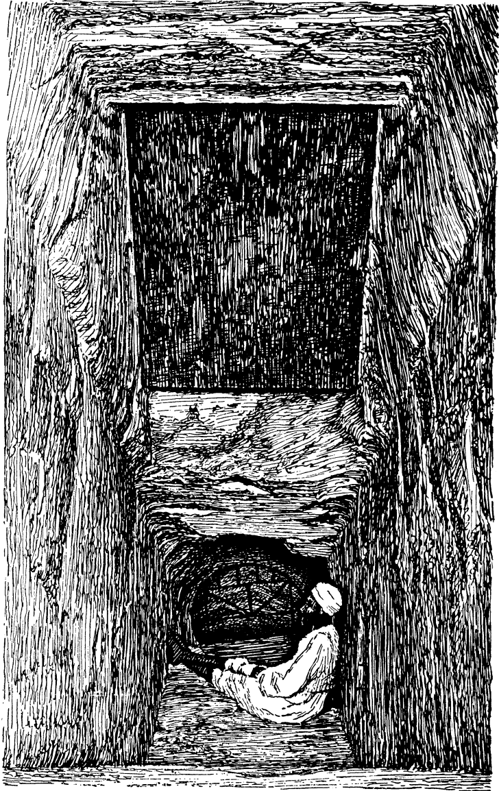
Depression in the roof of the Descending Passage of the Great Pyramid of Gizeh, showing the rectangular granite block, namely, the lower butt end of the Granite Plug
